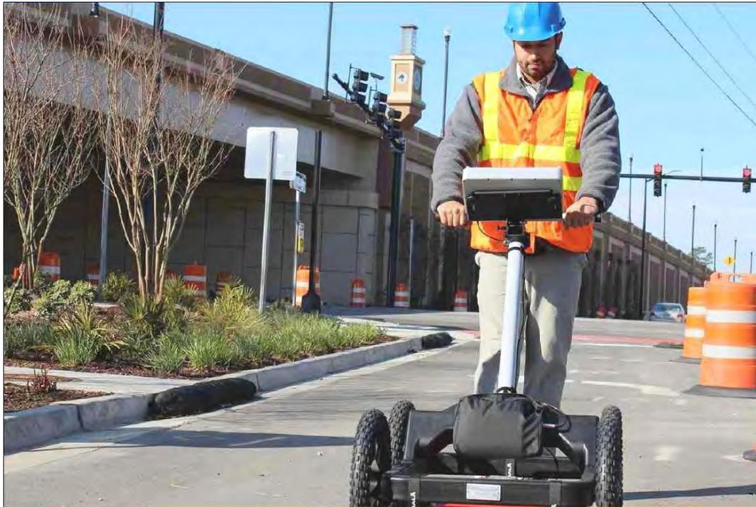
Advances in the design and construction of buried utilities have resulted in the ever increasing use of non-metallic materials. Locate professionals know the difficulties associated with non-metallic utilities and that conventional locating tools are insufficient in finding them. Ground penetrating radar is the only technology available that neither requires a physical connection to the utility, or the need to rely on its electromagnetic (EM) radiation.
